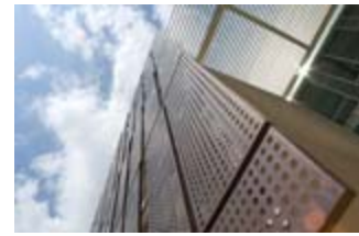
Marcus Nanotechnology Building at Georgia Tech formally dedicated — [24 Apr 2009] — Three years after breaking ground, Georgia Tech is set to dedicate the Marcus Nanotechnology Building, one of the most ambitious...
